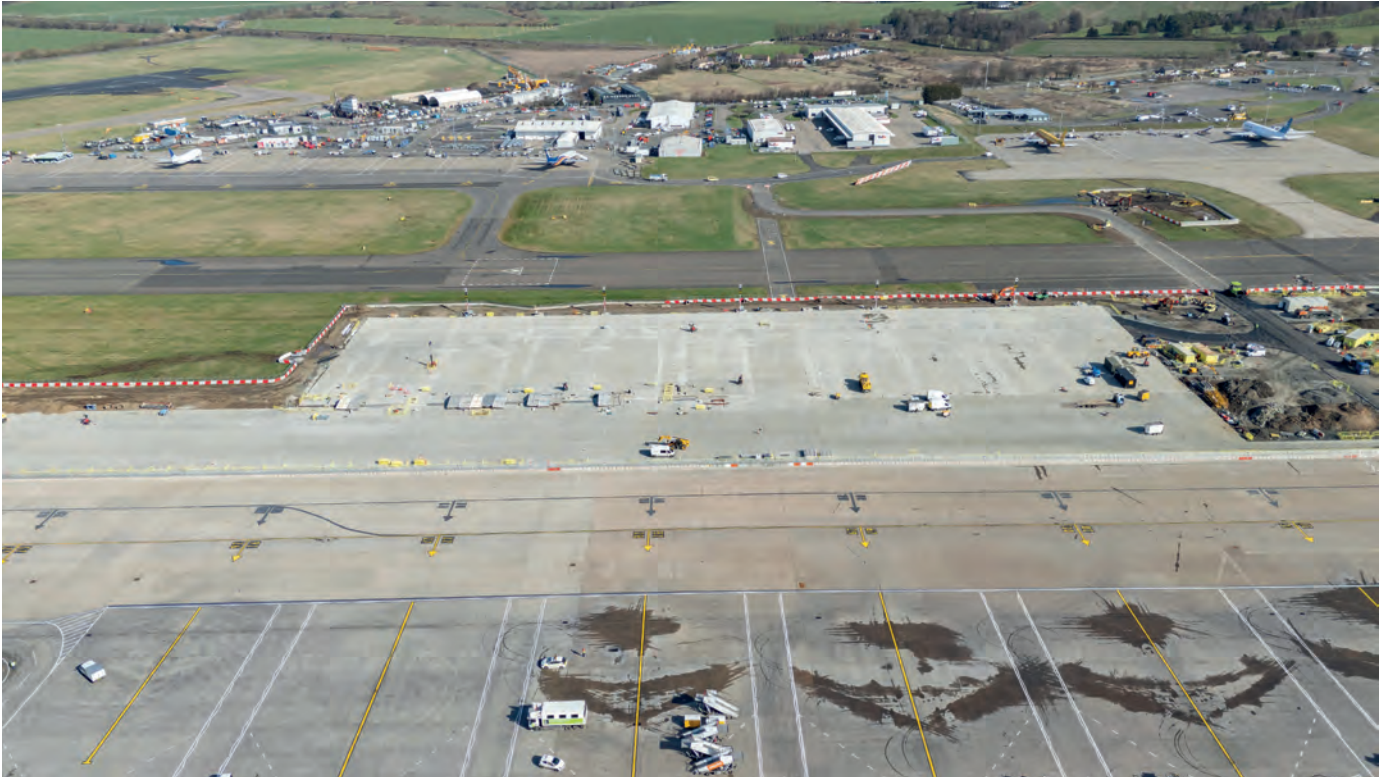
ABOVE: Midfield Stands project as works near completion.
