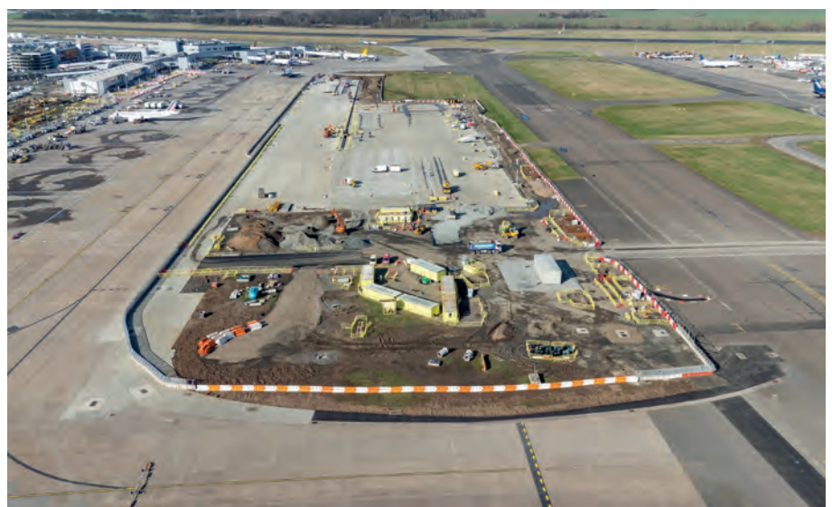
BELOW: Midfield Stands project mid works.
