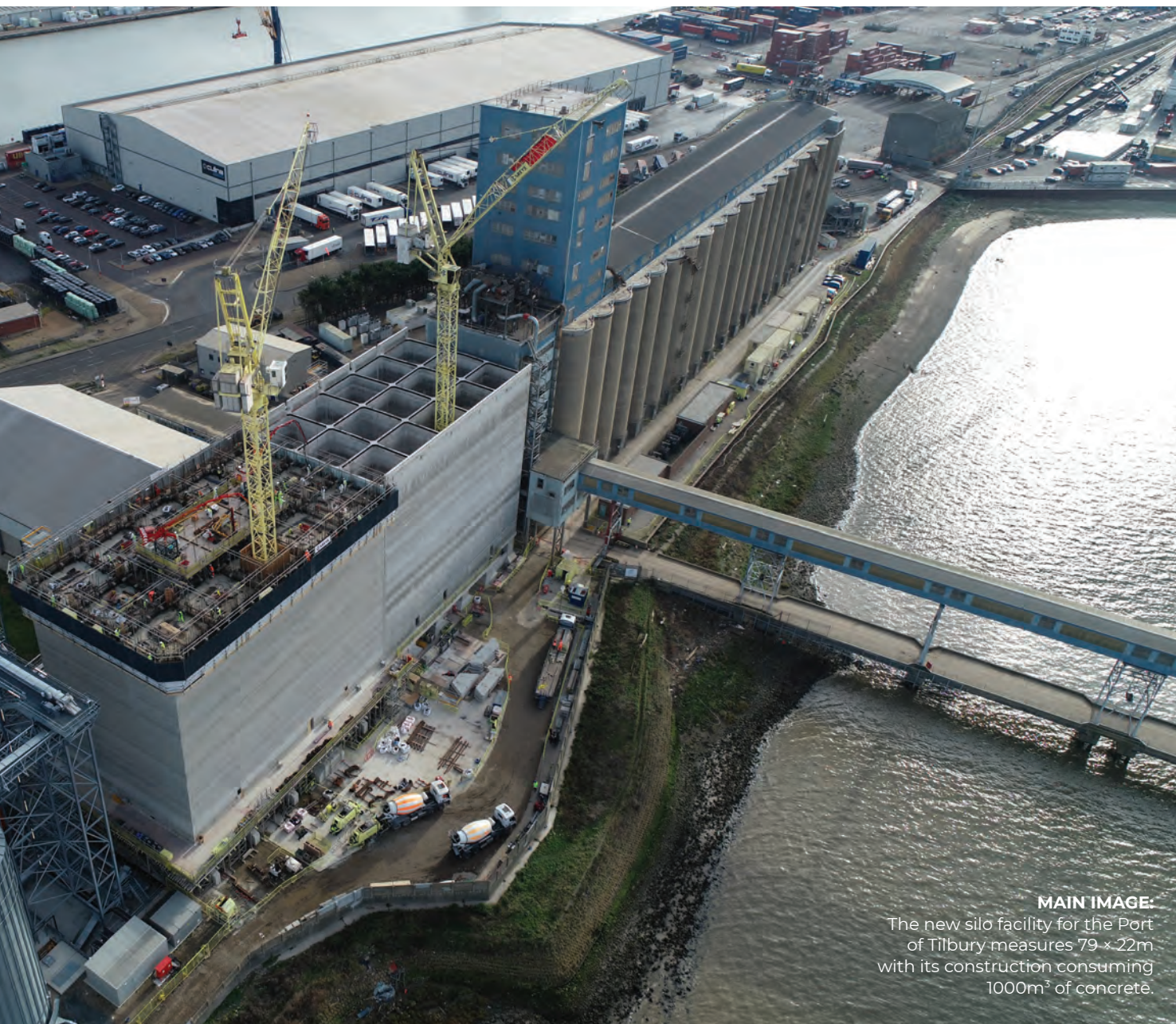
Gleitbau supplied a modified version of its well-proven, two-level slipform rig.
